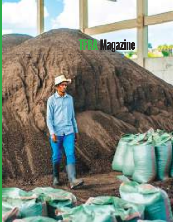
Mabwepande Composting Facility
